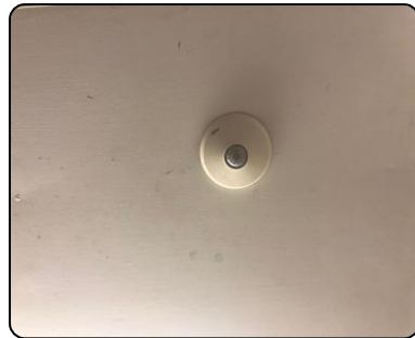
Motion Control Sensor for Rest Room Lighting
