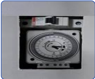
Timer Based AHU Operations Control
